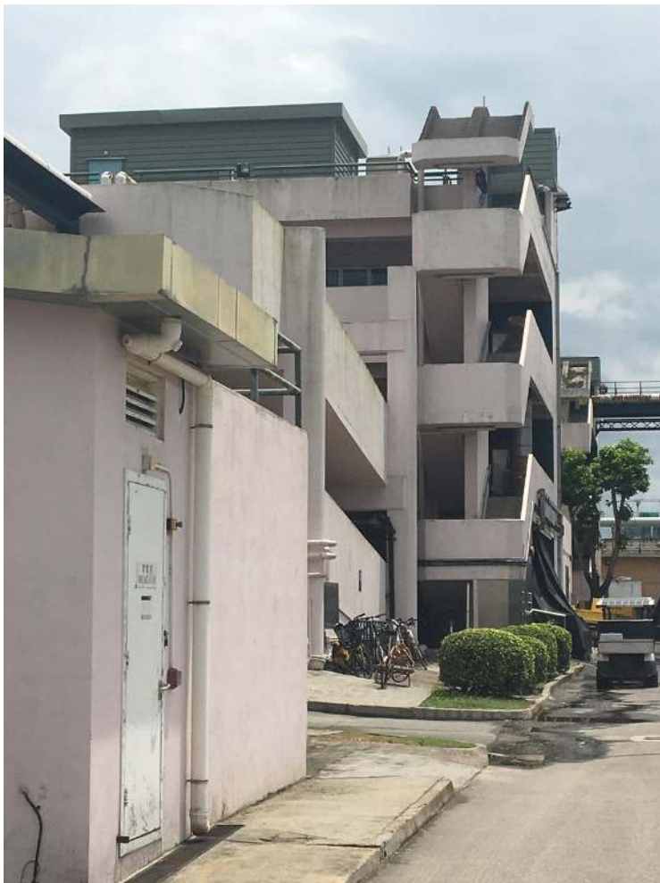
Four storey horse stable with ramps at KH Jockey Club
